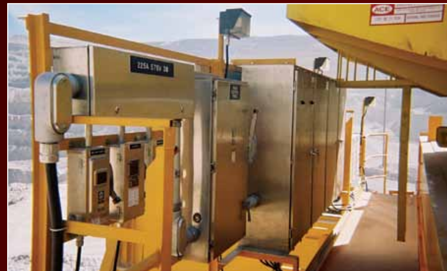
Custom controls for outdoor crane
