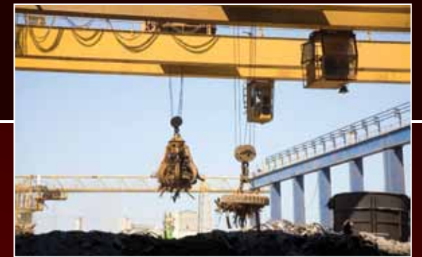
Scrap Handling Crane
