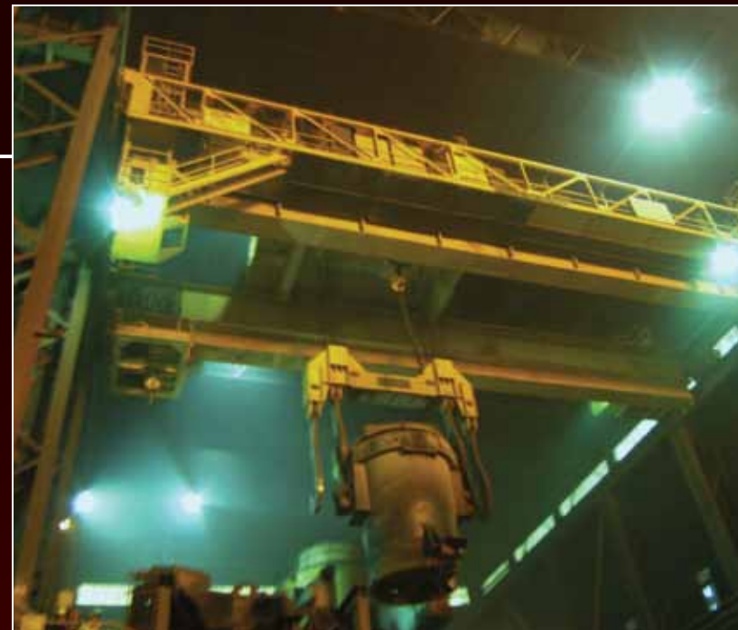
210-ton Ladle Crane with 60-ton Auxillary Hoist
