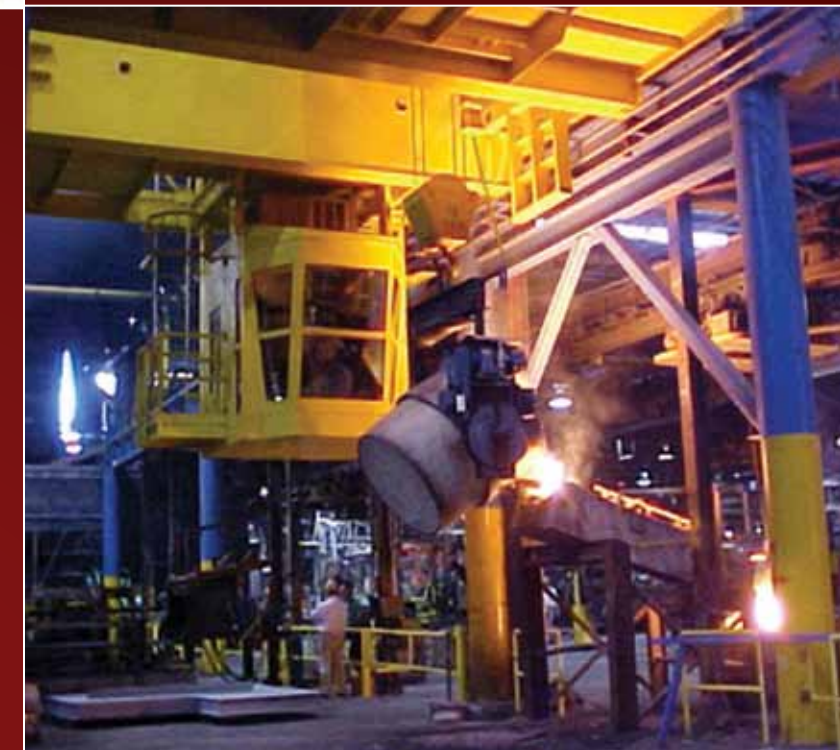
30-ton Ladle Crane with 10-ton Auxillary Hoist
